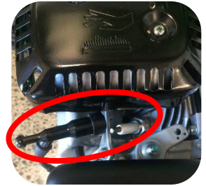
Disconnected spark plug
